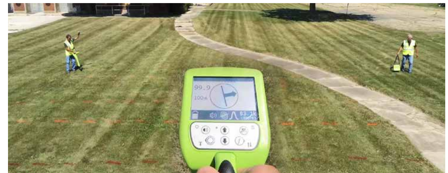
Figure 9: A Two-Man Sweep being performed to locate multiple parallel utilities.
