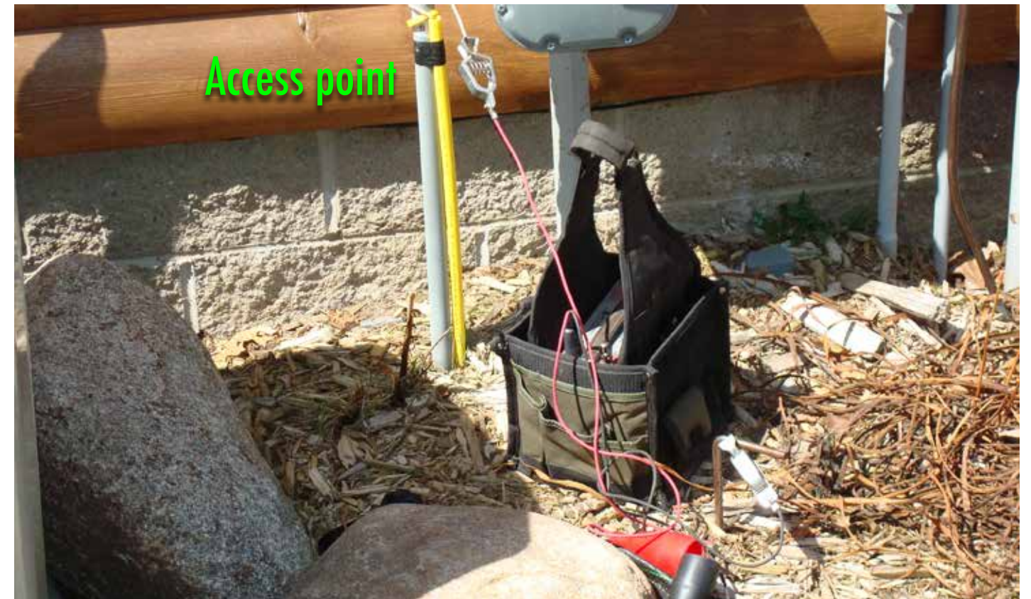
Figure 18: A connection to a copper tracer wire on a plastic gas service.
