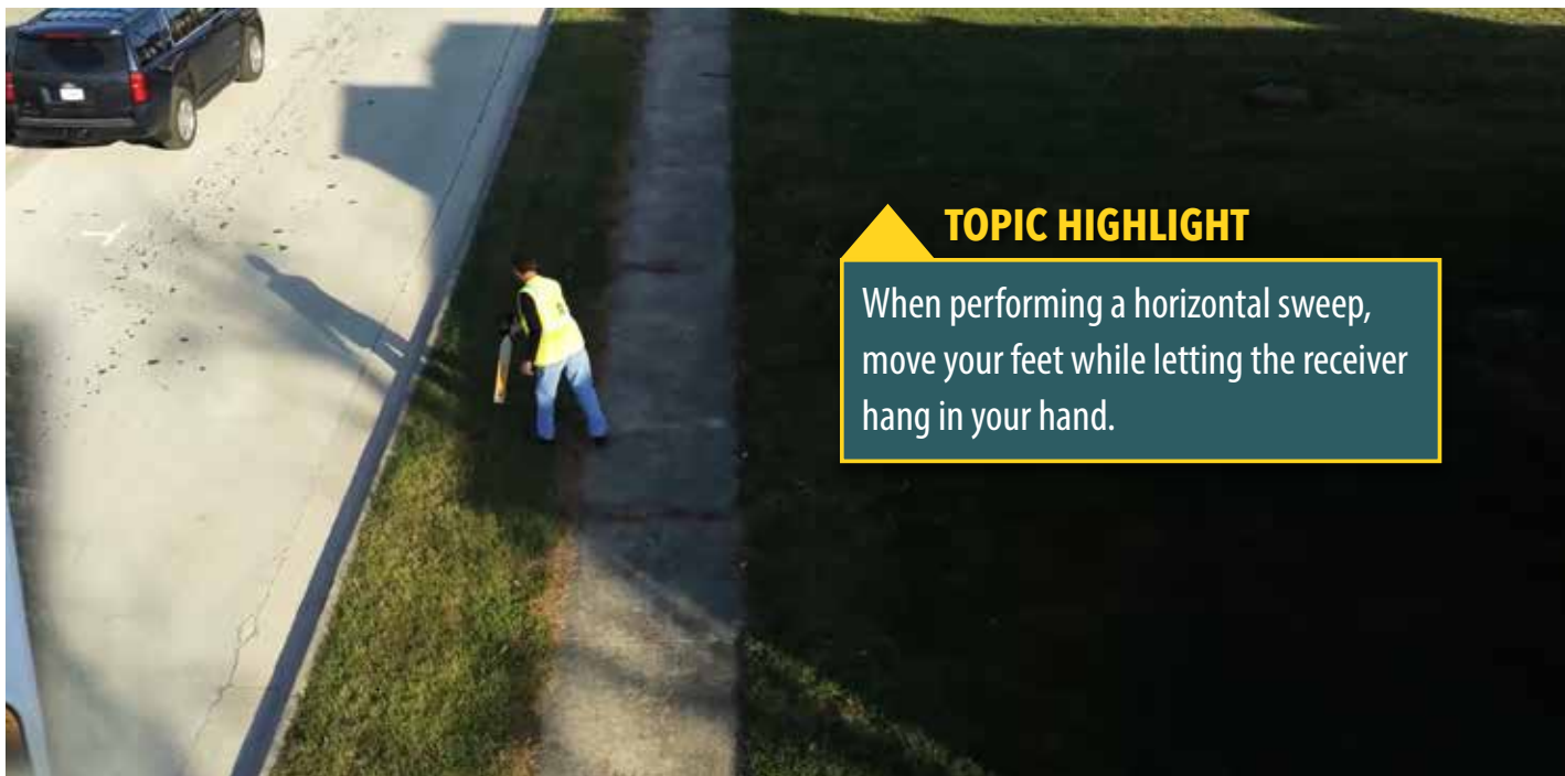
Figure 57: It's good practice to occasionally do a horizontal sweep across the right-of-way to make sure you're still on the target line.
